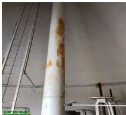
Corrosion at Base
