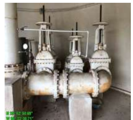
Corrosion at Base
